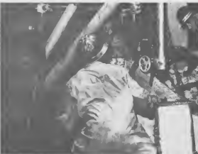
RIGGERS USE a chain block to remove a three-ton chunk of steel from the foundation of No. 5 Combination Unit, left. A hole is cut, center, to aid in rigging a block and tackle assembly. Nasario Tromp, metal trades foreman, right, inspects progress of the dismantling.
